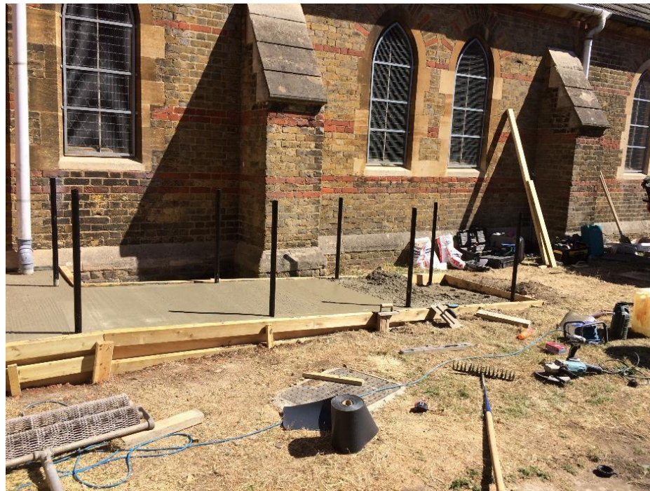
Emergency exit ramp under construction
