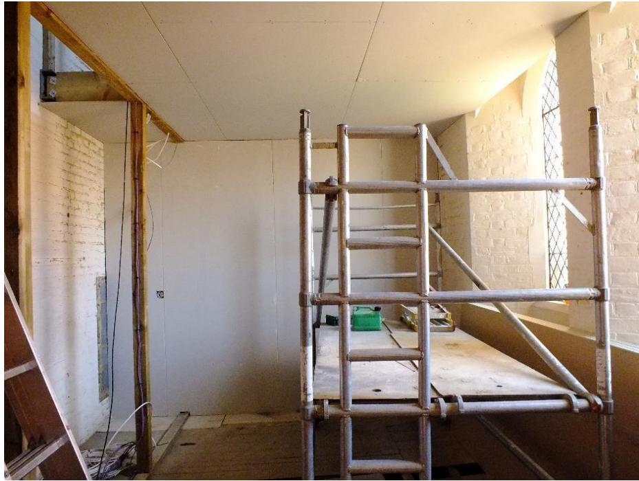
Plaster boarding of walls and ceilings
