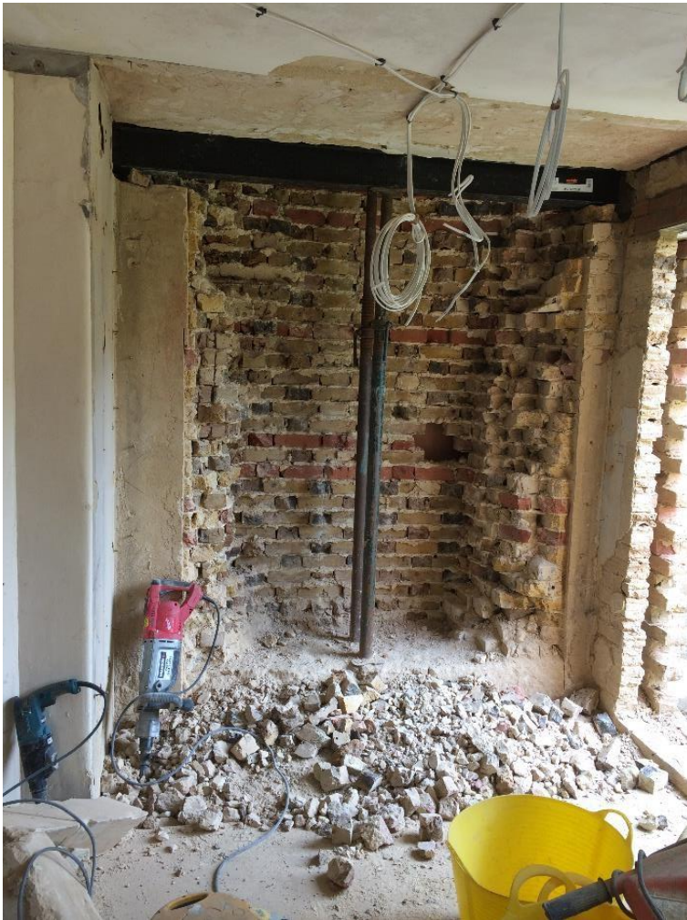
Cutting through the 700mm thick wall for the new doorway.
