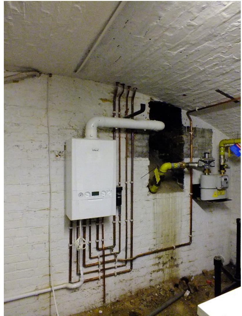
And new boiler installed
