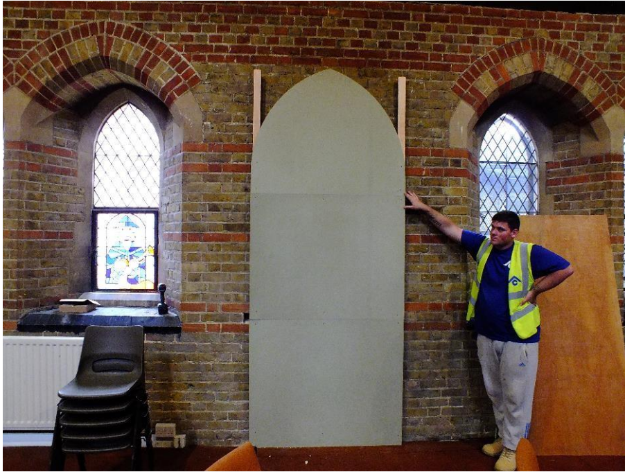
Checking the door shape is correct.
