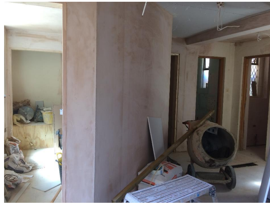
Followed by plastering
