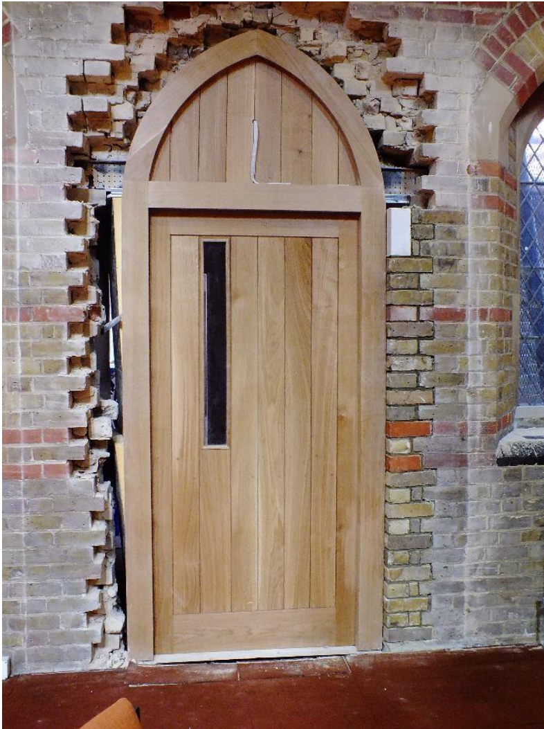
The oak door being installed
