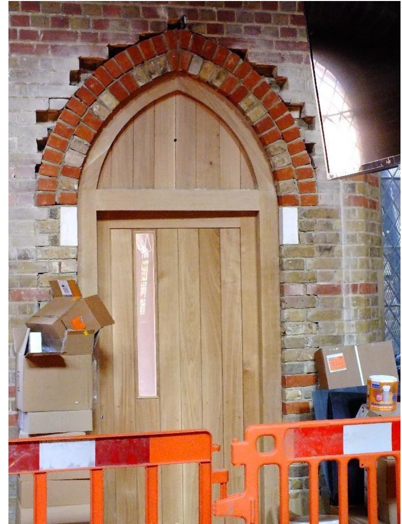
The arch brickwork completed
