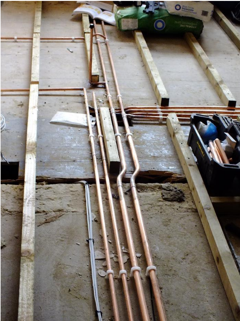
The plumbing is underway
