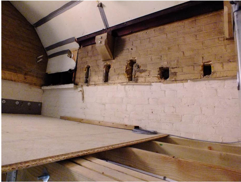
The mezzanine floor is laid
